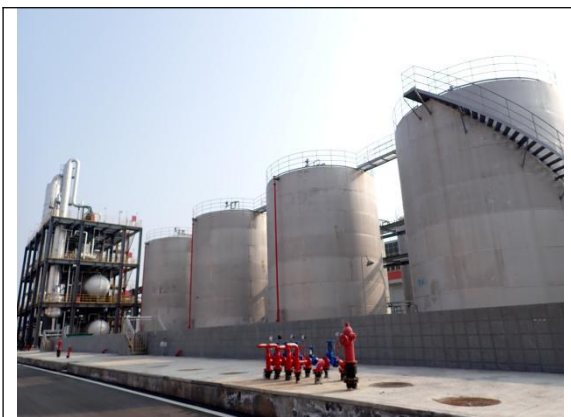
NMP 罐区围堰
